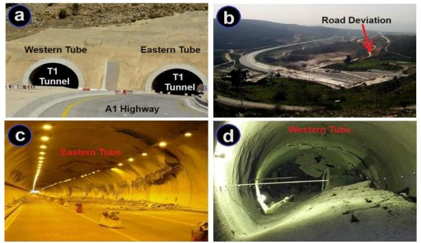
Figure 1. (a) Western Entrance of Tunnel T1. (b) Mountain bypass of the A1 highway route.(c) Partial collapse of the Right Tube (East). (d) Total collapse of the Left Tube (West).Source: Berkane et al. (2022), COSIDER SPA, Highway Management Agency (AGA).
