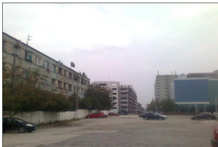
Figure 11. Social segregation in the urban physiognomy (leftside image: workers’ blocks of flats built in the 1960s-1970s mostly for single persons, in response to the development of an industrial zone in the west of Bucharest city; presently, it is low-income families that live there; rightside image: “West-Gate”, a new residential and business quarter developed after the year 2000, inhabited by families with over-average incomes. Note: separated by a concrete wall) (Source: author, 2018)
